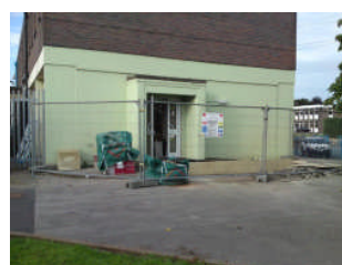
Flint High School - external ramp works
