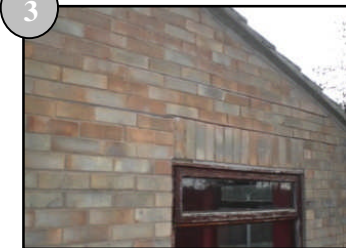
3 Slot cut for masonry beam above window and soldier course ties.
