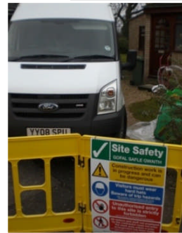
The H&S fencing and signage onsite
