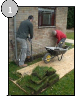
1 First step is to prepare the trenches.
